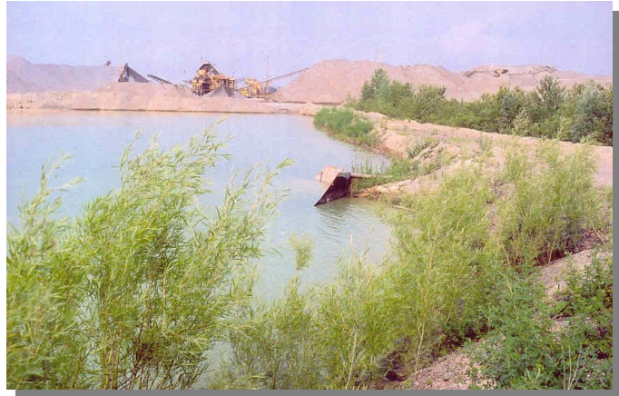
Settling ponds are used to collect water for recycling
