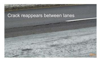
Figure 35. Highway 427 – Reappearance of Cracks Between Lanes in 2011
