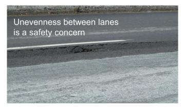
Figure 36. Highway 427 - Pavement Distresses Between Lanes in 2010 - 2011
