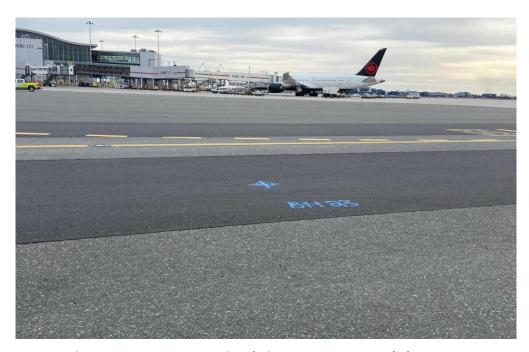
Figure 15. Pearson International Airport – T1 Apron Asphalt Observed Patches in Fair Condition (EXP - November 2021)
