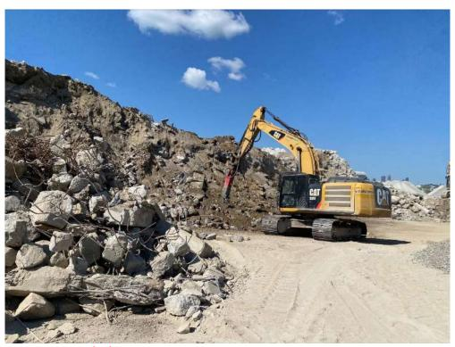
Photo (31): Strada Aggregate Crusher: 10 Leslie St, Toronto, ON Breaking Big Pieces of Concrete Prior Crushing
