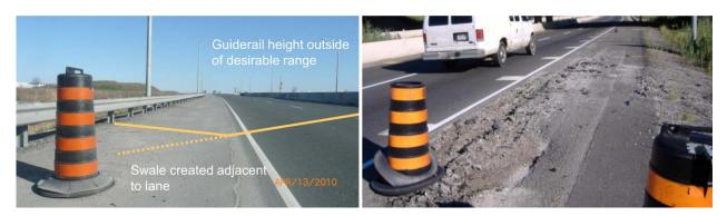
Figure 37. Highway 427 – Guiderail Height Outside of Desirable Range and Swale Created Adjacent to Lane (2010)
