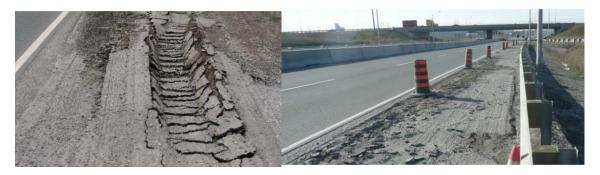
Figure 38. Highway 427 - Different Pavement Distresses (2010 -2011)
