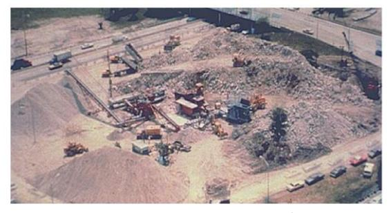
Figure 22. Concrete Recycling Operation Set up Inside of Edens Expressway Cloverleaf Interchange (Photo from NHI 1998) [13]
