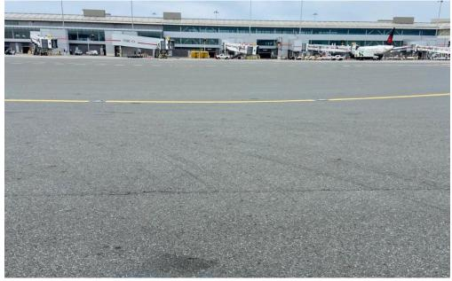
Figure 16. Pearson International Airport – T1 Apron Asphalt, Occasional Construction Joint Cracking in Slight to Moderate Severity.
