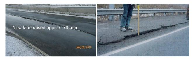
Figure 34. Highway 427 – Pavement Heaving in 2010
