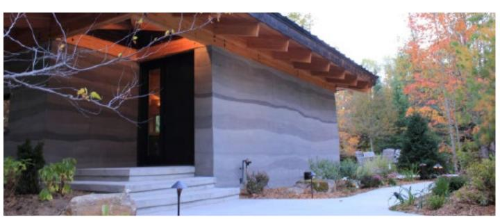
Tapial Homes uses a rammed earth mix comprised of 90 per cent locally sourced aggregates for its homes. Photo courtesy of Sprout Studios
